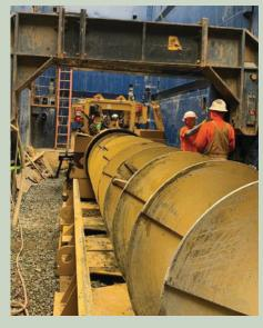
be done using auger boring from cost, safety and timeframe perspectives. Other trenchless methods such as horizontal directional drilling (HDD) and microtunneling were ruled out due to the depth of the bores and space limitations at the site.
